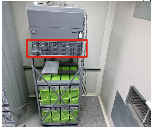
Solar subrack with DC solar converter (right):
